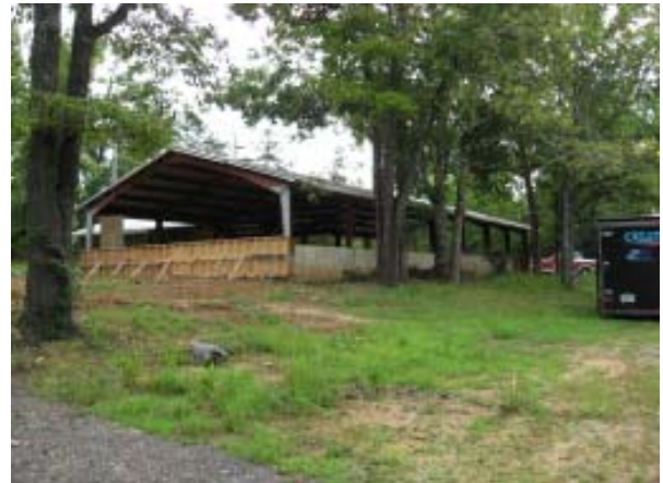
Dining Hall with concrete forms in place
