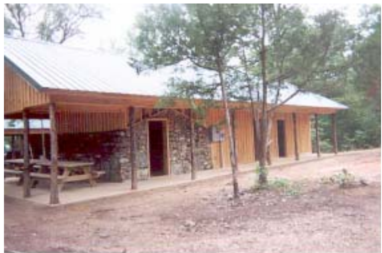
Office, Walk-in Freezer and Storage Building
