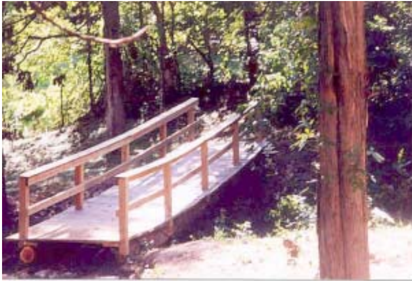
Foot Bridge over Spirit Creek
